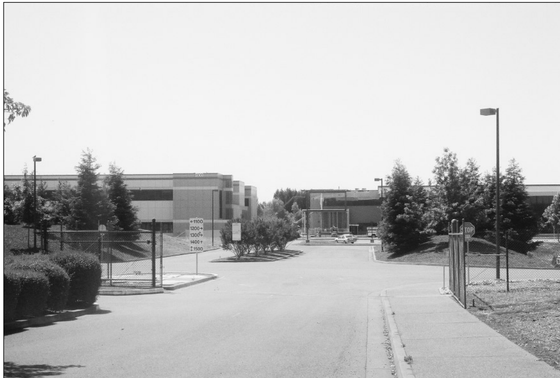
B. VIEW SOUTH INTO PROJECT SITE AT NORTH ENTRY.
